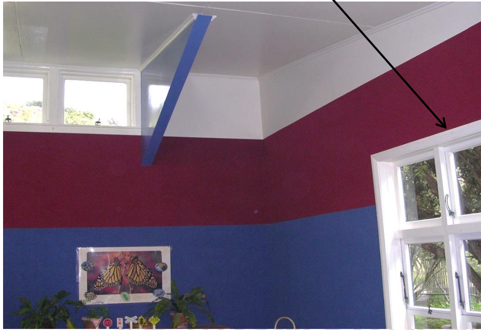
Figure 7a Acoustic composition wall panels applied to the wall surfaces in a New Zealand kindergarten
