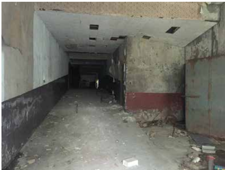
Figure 2. Entrance to the cinema halls of Fu He Grand Theater. Author's photo, May 10, 2016.
