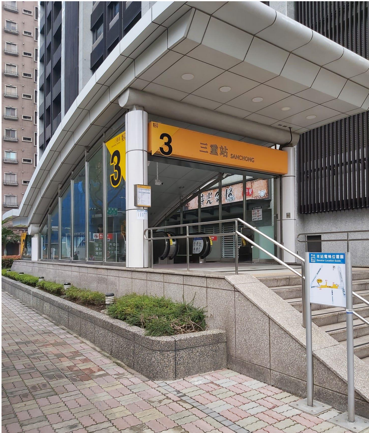
Figure 1 - Typical Taipei Metro entrance, New Taipei City.
